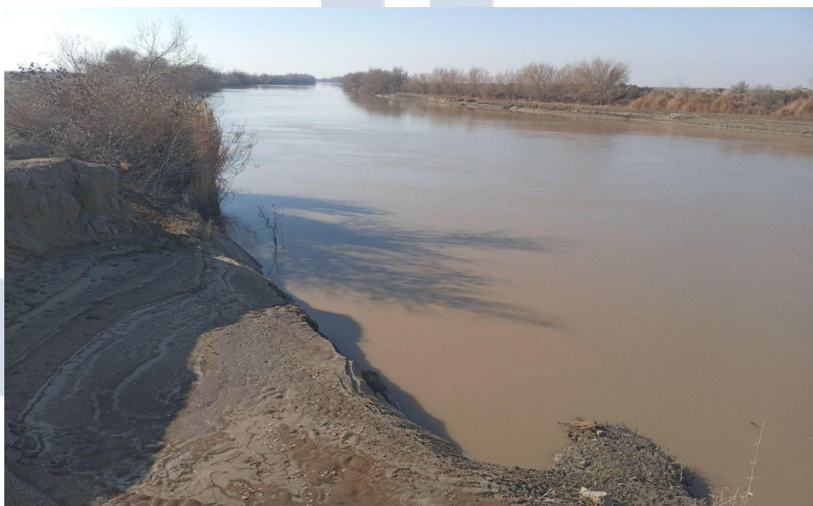
1-2- rasm.Guliston-Namgon kanalining qirg'oqlarining yuvilishi
