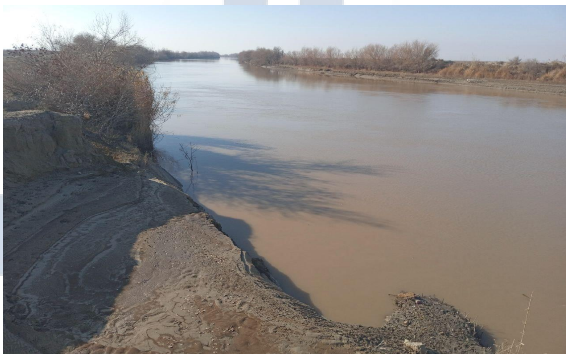
1-2- rasm.Guliston-Namgon kanalining qirg'oqlarining yuvilishi
