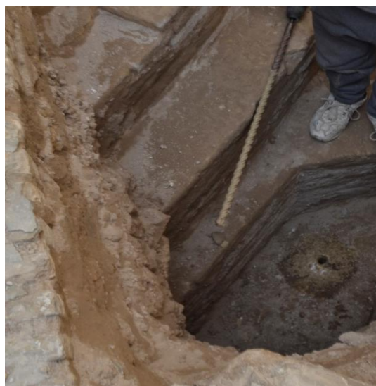
Figure 2. The process of studying the foundation of the minaret by Islom Khoji
