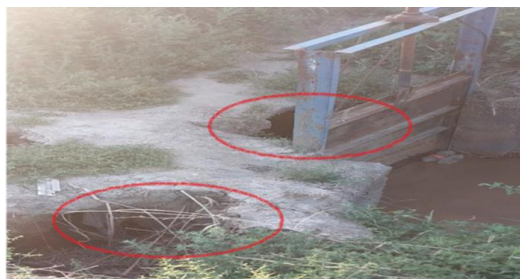
4-rasm. Arabi kanalining hozirgi paytdagi texnik holati
